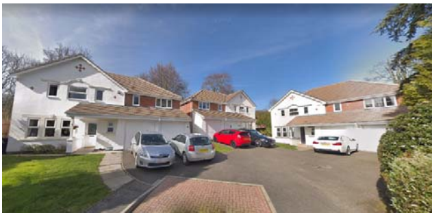
View of existing dwellings within Ruxton Close
